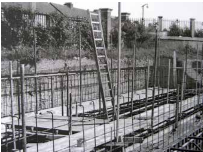
The bunker under construction in 1953.
